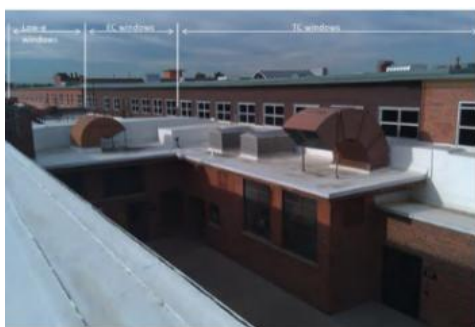
Figure 2. Exterior view of the west façade showing the locations of three types of windows. Low-e windows were installed in 2005. [16]
