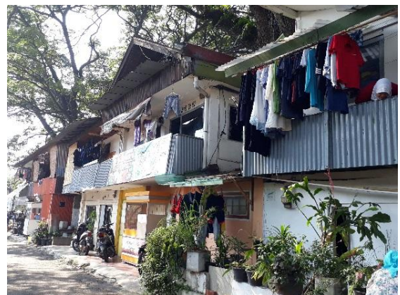
Figure 7. Balcony configuration and height on the Jongko house
